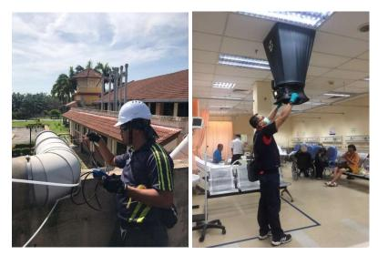
Figure 14.11. Inspection, testing and examination of ventilation system
