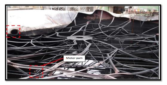
Figure 10.6. Condition of the manhole (maintenance location) and pump motor the remaining RFO
