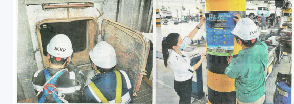
DOSH officers inspecting a confined space at a Tenaga Nasional substation in Marang. (R) DOSH officer (standing behind) with a car service centre staff placing a workplace safety and health poster.
